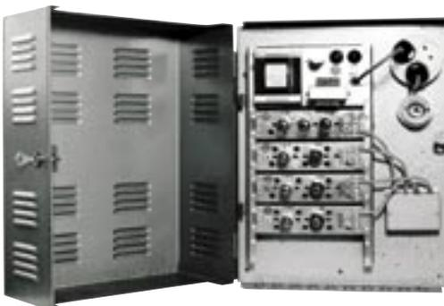
**An antenna amplifier centre**, which could be found in the basement or attic of most Finnish apartment buildings.
